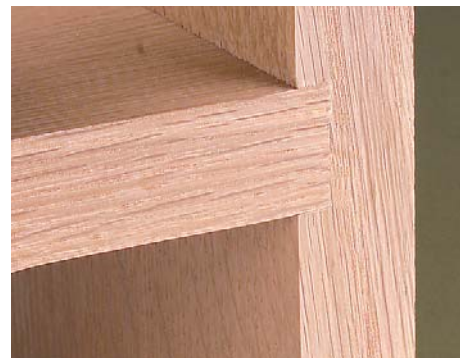
▲ Best. To get the tightest, best-looking dado joint, use a dado clean-out bit in a hand-held router. The top-bearing bit is guided by the sides of the dado.
